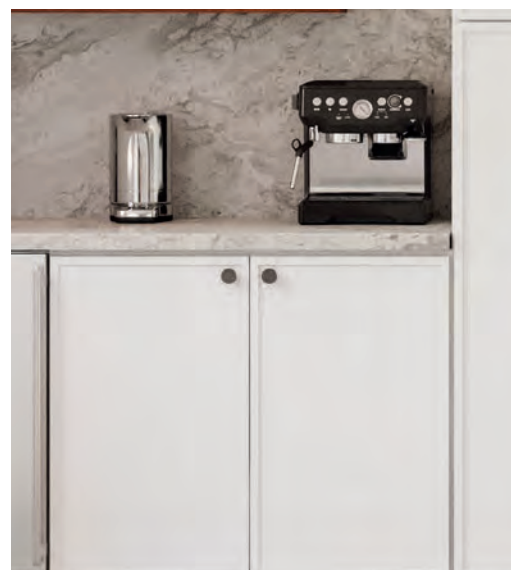
Wall cabinet modified to a base cabinet
